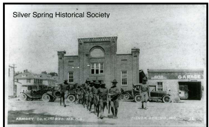
1914 Armory in Silver Spring, remodeled as a fire station in 1927
